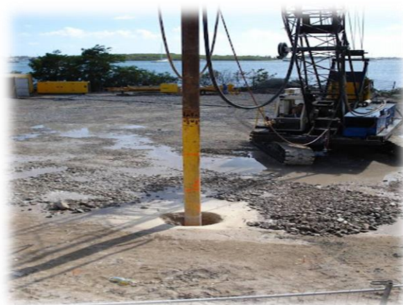
Figure II.2. Le vibro-compactage
