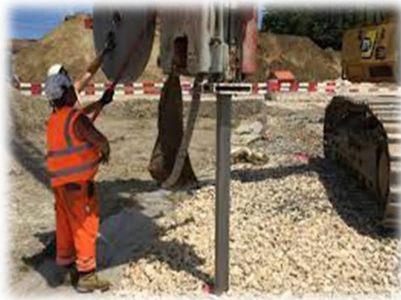
Figure II.3. Installation des drains verticaux
