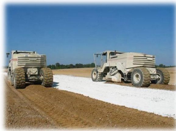
Figure II.5. Application des liants hydrauliques routiers
