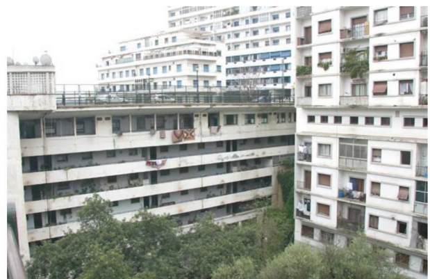
Figure 64: immeuble pont / source: www.mutualheritage-alger.univ-tours.fr
