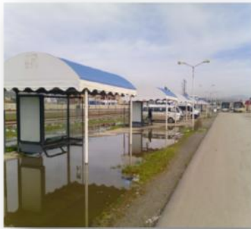
Figure 76: abri bus inondé
