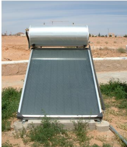
Figure. I.20 : chauffe-eau solaire monobloc.
