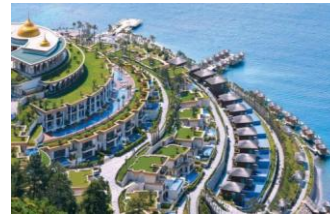
Fig. 4.23. Architecture et Mer Source. The Plaza Bodrum
