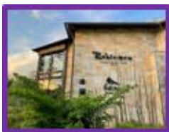
Fig. 3.53. Restaurant Robinson Source. Google earth
