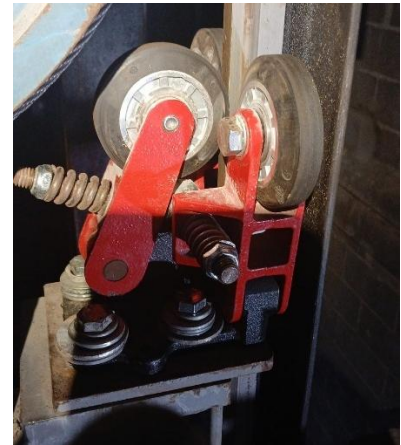
Figure II-15 : Roller guide.
