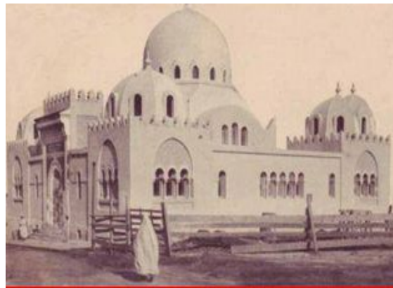
Figure 33 : Djamaa Abderrahmane. Source : PPSMVSS.
