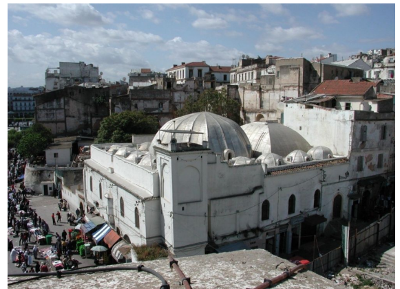
Figure30: Djamaa Ali Betchine. Source : PPMVSS Alger.
