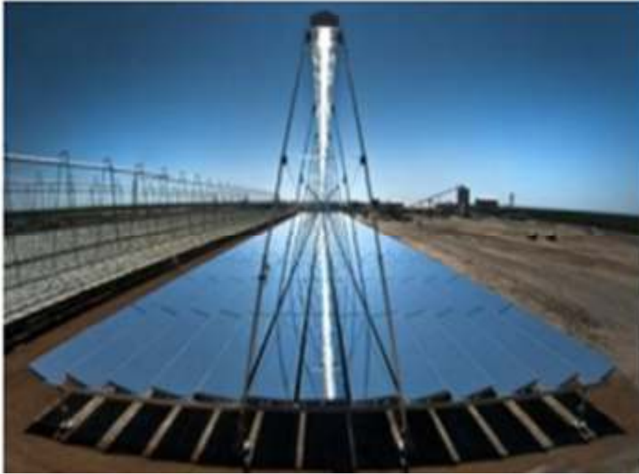
Figure II.6 : centrale solaire a miroirs de Fresnel [22]
