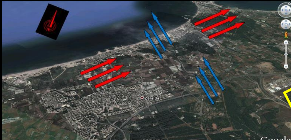
Fig29: les vents dominants SS: image satellite (Google earth)
