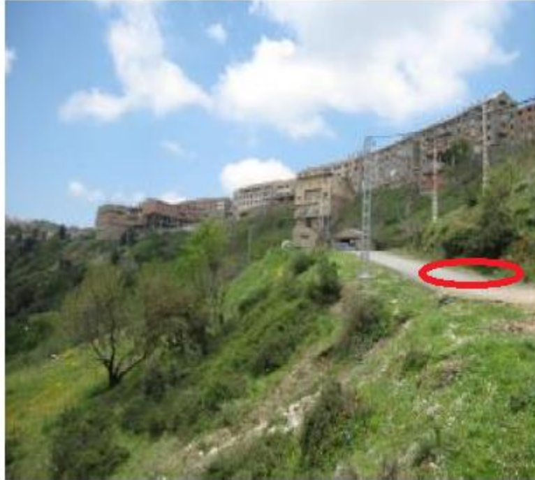
Figure II-22: affaissement de la route (source: Djerbal,2010)
