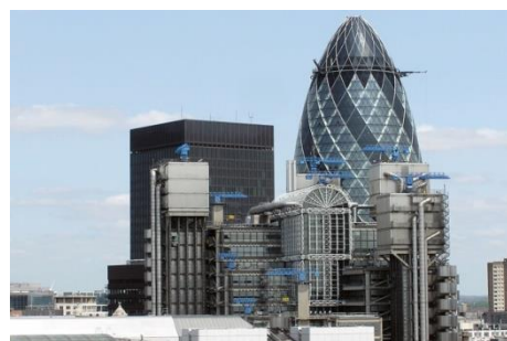
Figure 95 : le Lloyd's building, Londres Source : https://en.calameo.com
