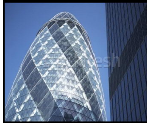
Figure 1: tour Swiss Re Londres Norman Foster http://www.building.com.uk
