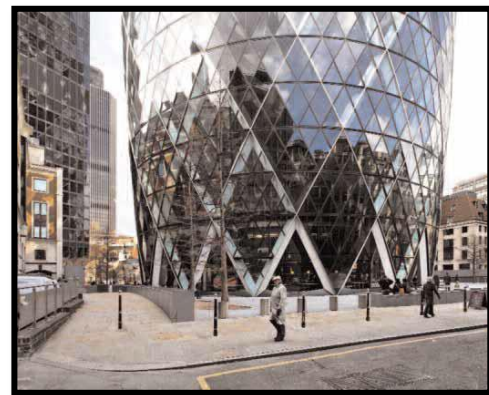
Figure77: structure V inversé. http://www.constructalia.com
