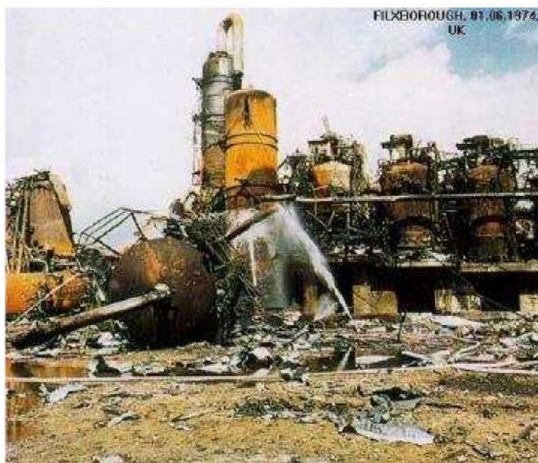
Figure 2.1: Accident de Flixborough, UK (1974) [27].
