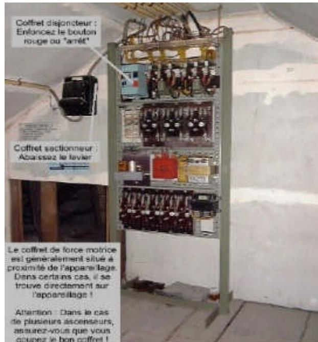
Figure I- 18: Coffret de force motrice.
