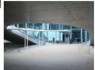
Figure 117 : Entrée Est. Source : www.concrete-hub.com
