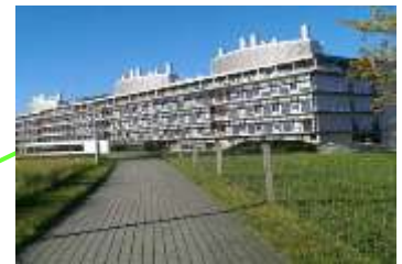
Figure 107 : UNIL- Batochime. Source : Google earth, street view.
