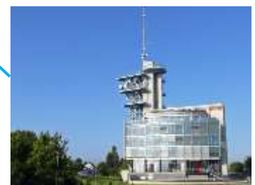
Figure 105 : EPFL EMBA Program. Source : google earth, street view.
